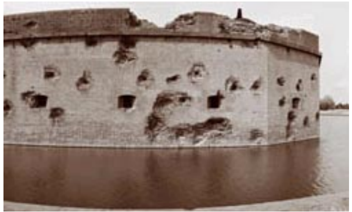
Today the unrepaired effects of the bombardment can still be seen.
